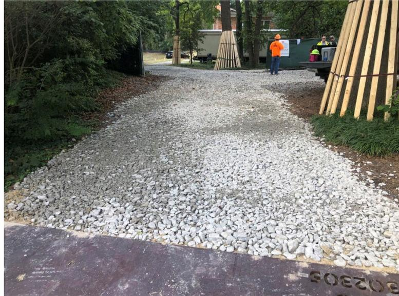
New stone in place for the stabilized construction entrance plus tree protectors installed along the access road
