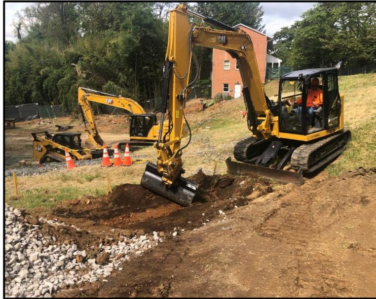
Excavating Eastern Drainage Swale for erosion control
