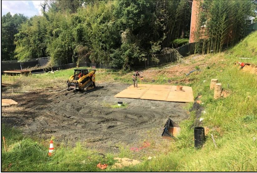
Installing poly Construction Mats within the former PSB footprint to protect the clean backfill & stabilize surface for excavation operations
