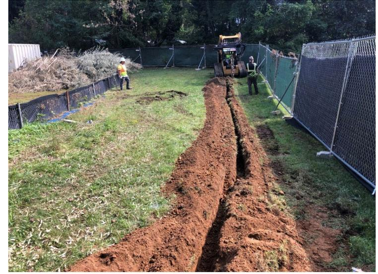
Excavating anchor trench for the Super Silt Fence to be installed within the limit of disturbance along the southwestern edge of the site
