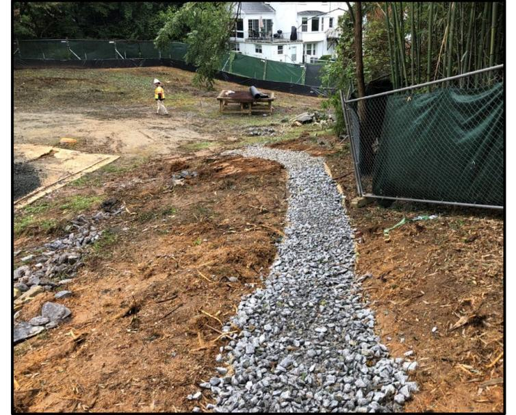
Completed Western Drainage Channel for erosion control and New Super Silt Fence at back
