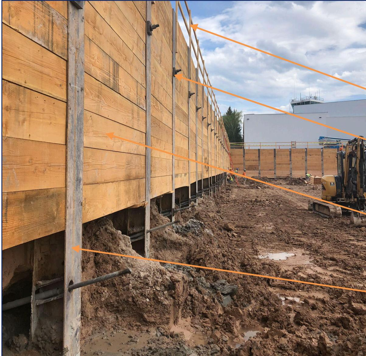
**Install ~14 ft Retaining Wall from elevation 362 ft down to 348 ft and excavate approx. 560 CY of Debris**
